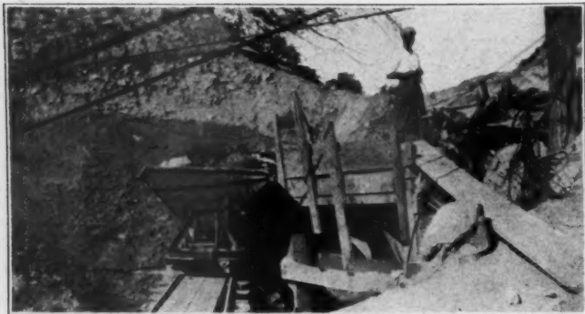
Dump Car Carrying Cobbles from Grizzly to Waste Pile. Little Falls
